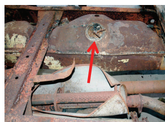
The failed muffler (bottom) and fuel tank (top) with arrow indicating where the truck’s plastic fuel lines entered the tank and were melted by hot gases and flames from the failed muffler.
